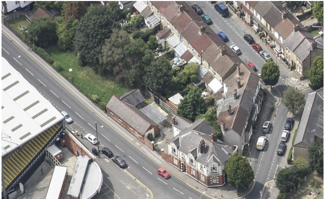
Fig. 2. Aerial view of site.
